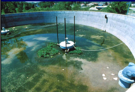
Leeds, AL, wastewater treatment plant, SSO storage tank
