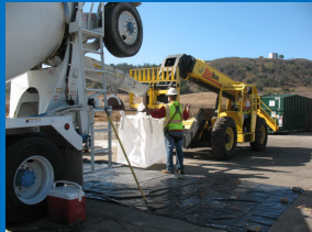
Filling individual media bags prior to mixing
