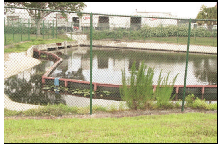
Settling Pond after Alum Injection, Orlando, FL
