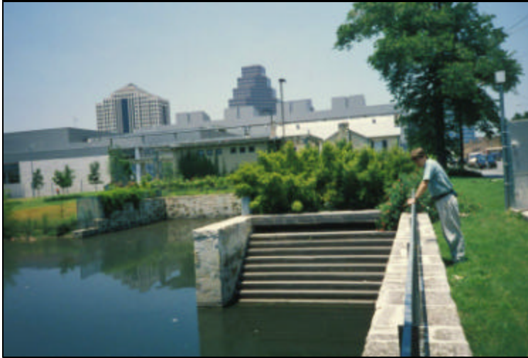
Wet Pond after Oil and Grease Trap and Step Aerator, Austin, TX
