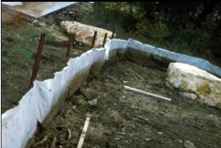
Filter Fabric at Construction Site Showing Maximum Water Depth
