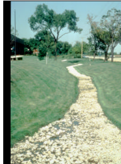
Infiltration Swale in Office Park Area, Downstream of Wet Pond, Lake Oswego, OR, Part of Treatment Train
