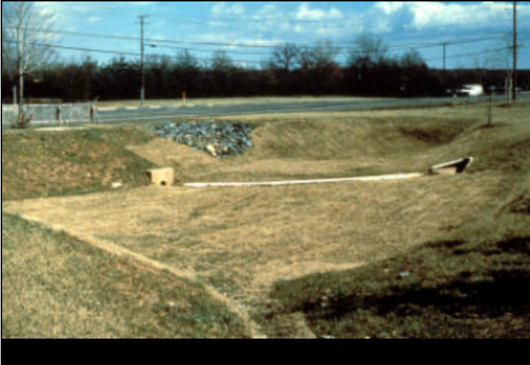
Typical Dry Detention Pond, with Pilot Channel
