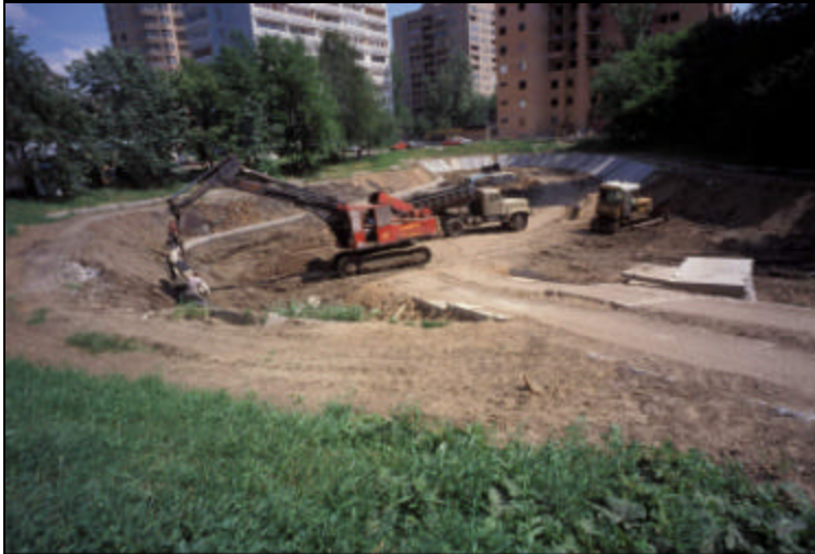
Re-building Pond (Re-shaping and Dredging), Moscow, Russia
