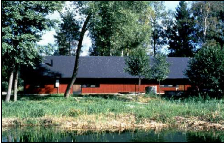
Ferric Chloride Treatment Unit at Lake Ronningsjön, Taby Sweden (Karl Dunker)
