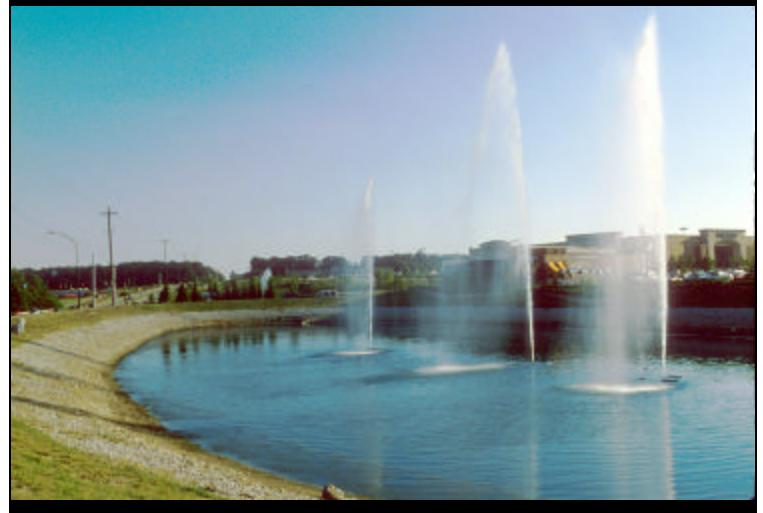
Wet Detention Facility at Shopping Center, Dayton, OH
