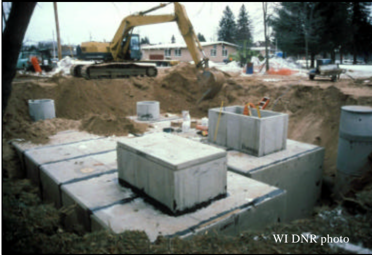
Backfilling MCTT at Minocqua, WI
