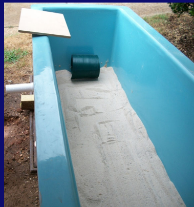
SmartDrain™ installation in the drainage sand (it was unrolled before placement of the cover sand).
