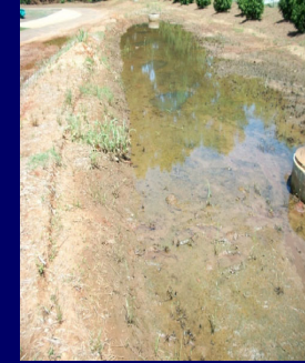
Extended ponding of water in low area of biofilter after rain.
