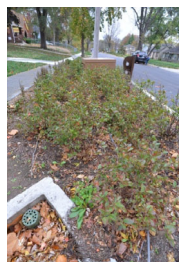
1324 76 th St. monitoring location, biofilter and adjacent porous concrete sidewalk (one of 10 monitored, along with the large-scale system monitoring of whole drainage areas)
