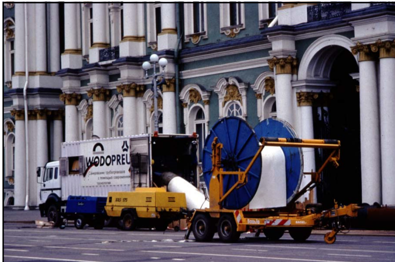
Re-lining of a large sanitary sewer to reduce infiltration.
