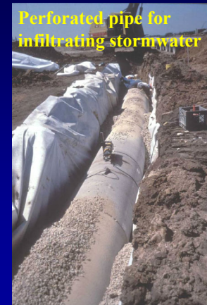
Older infiltration trench at parking lot
