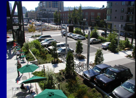
Portland, OR, site having green roof, porous pavement, and biofiltration
