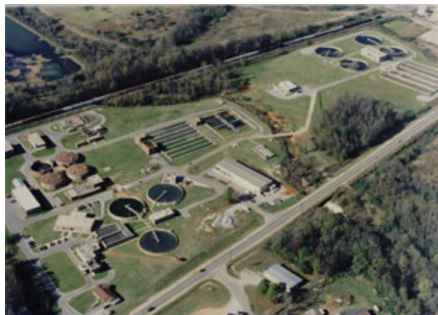
City of Tuscaloosa photo
