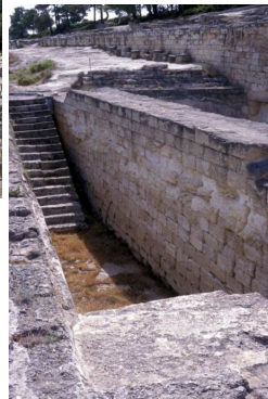
Jug-filling area next to cistern
