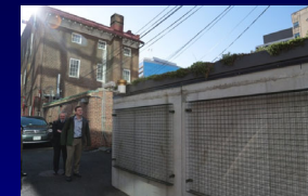
Water storage tank at Washington, D.C. fire station storing roof runoff.
