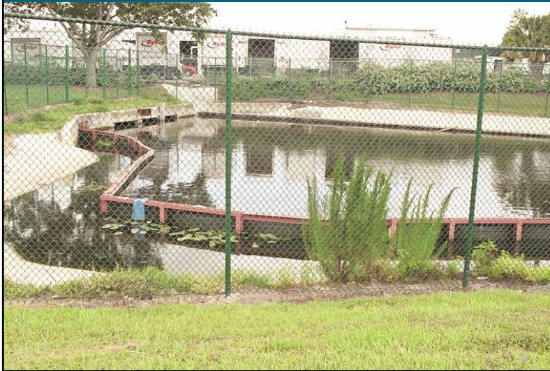
Settling Pond after Alum Injection, Orlando, FL
