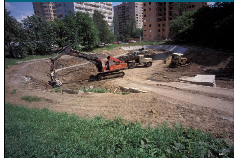
Re-building Pond (Re-shaping and Dredging), Moscow, Russia
