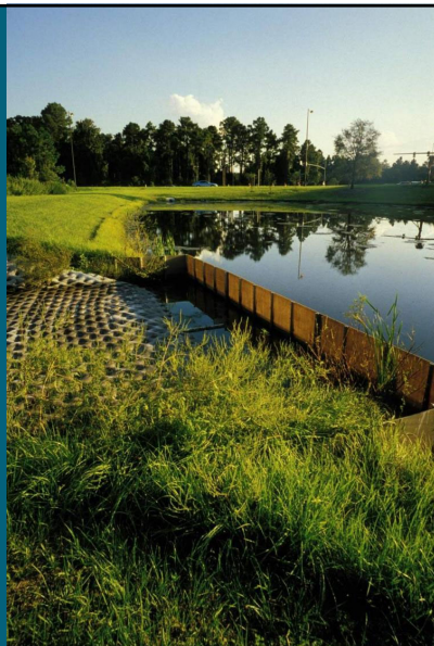
Modification of Pond Outlet at Epcot Center, Orlando, FL
