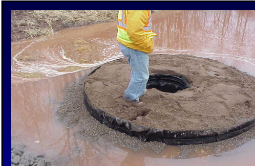
Turbid flow moving through the sand filter system, entering the perforated outlet pipe which discharges to a drainage swale offsite (D. Lake photo)
