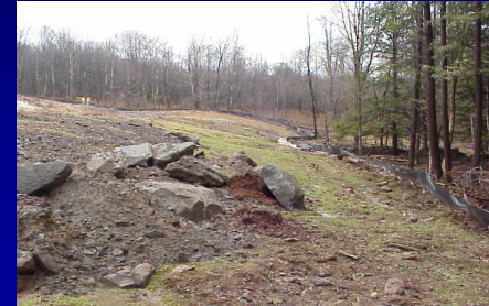
Excess excavation deposited in a forward cell of the waste area when haul road became impassable (D. Lake photo)
