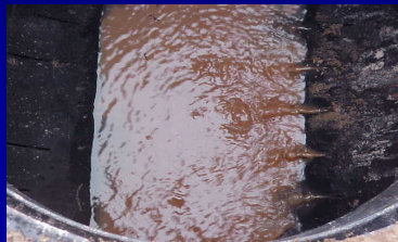
Turbid flow moving through the sand filter system, entering the perforated outlet pipe which discharges to a drainage swale offsite (D. Lake photo)
