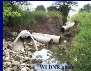
Even concrete-lined channels and pipes may fail
