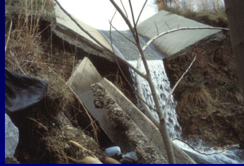
Even concrete-lined channels and pipes may fail
