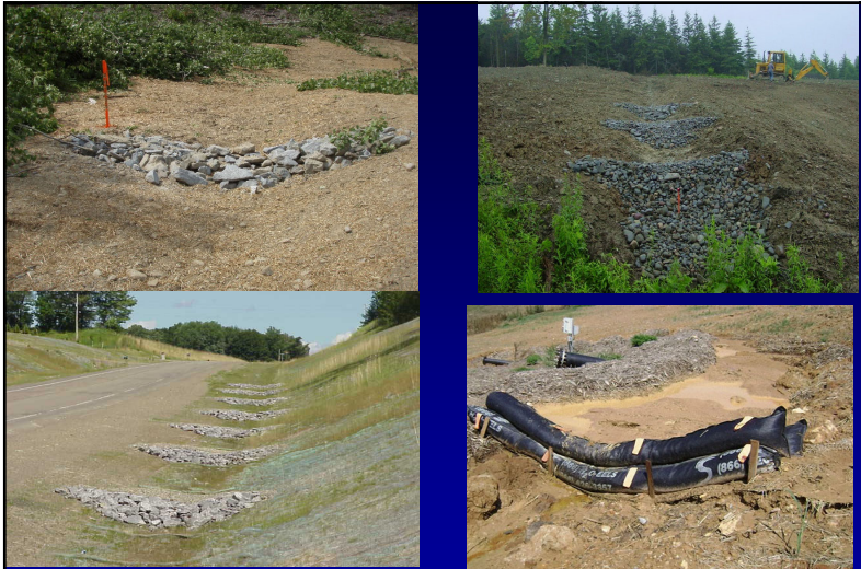
Check dams at construction sites (straw bales are no longer allowed by most US regulatory agencies as an approved control) 37
