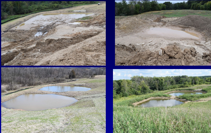
Sediment pond dredging, replanting, and final pond at construction site
