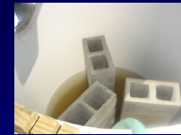
Installation of blocks to set the false bottom
