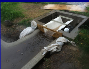
Influent from parking lot to flow splitters and test sections
