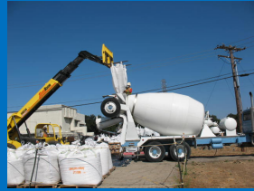
Loading media bags into mixer for blending media mixture
