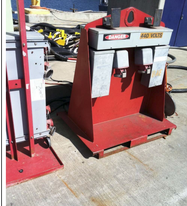
Galvanized metal circuit breaker boxes at naval base
