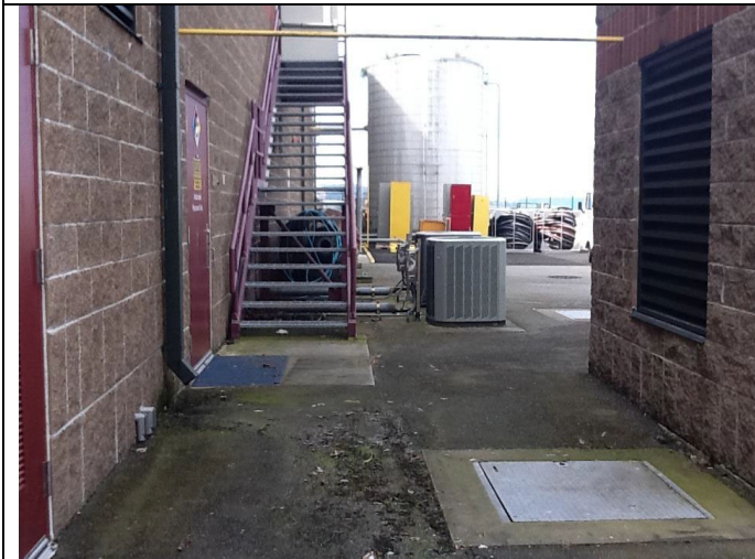
Galvanized metal stairway (painted) at naval base
