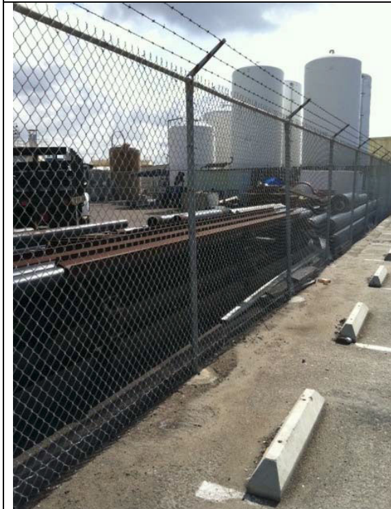
Galvanized steel fencing at naval base
