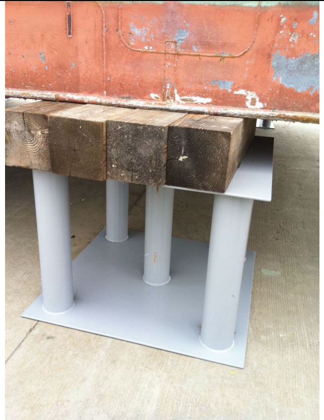
Medium laydown area, painted metal barge support stands, treated wood, and barge (on concrete) at naval base
