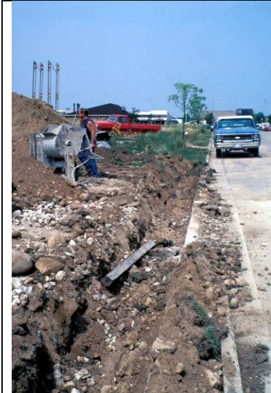
Utility work near street.
