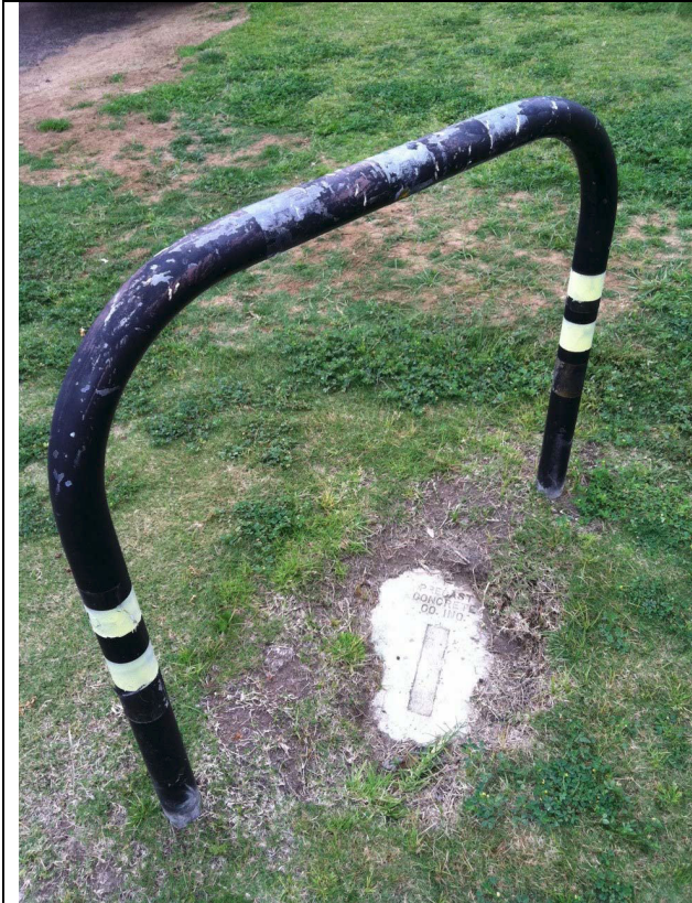
Galvanized metal pipe parking barrier at naval base
