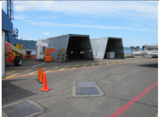
Galvanized metal roofs, galvanized storage sheds, drains to ground.
