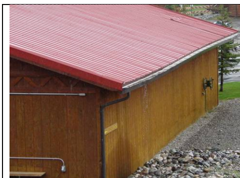
Pitched metal roof
