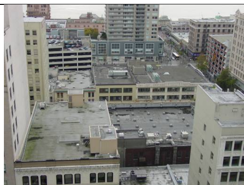
Flat commercial roofs
