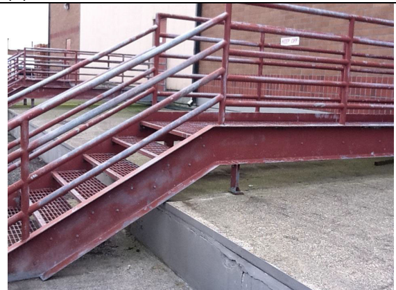
Galvanized metal stairway (painted) at naval base
