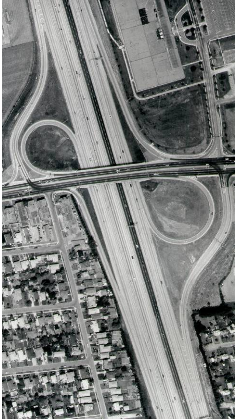
Example aerial photograph of freeway land use area (Pitt and McLean 1986).
