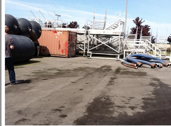
Heavy storage/laydown area, rubber bumpers, aluminum stairs/walkways, some galvanized materials, conex and hoses (on asphalt) at navy base
