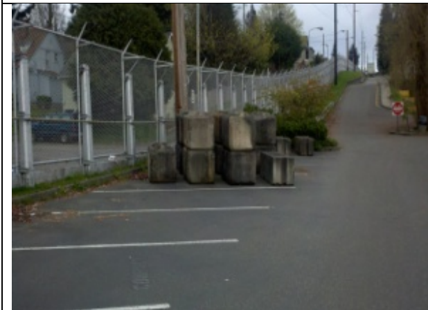
Fence, painted galvanized; NB Kitsap
