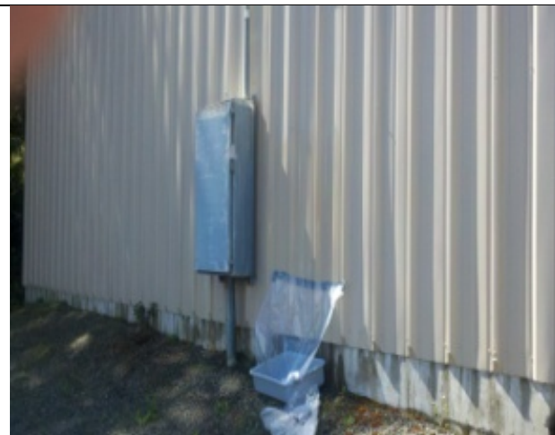
Metal panel, painted light yellow; Bangor
