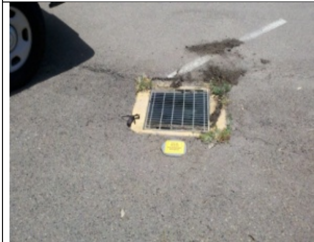
Grate 1, stormwater drain; NBSD
