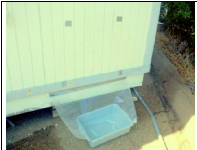
Wood wall, painted; SSC-PAC
