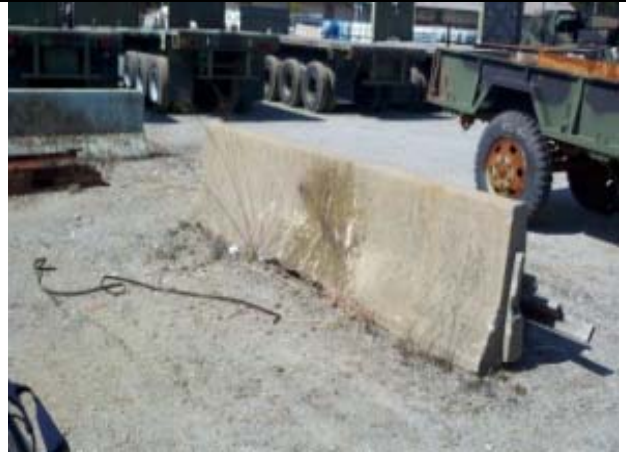
Concrete barrier, uncoated; Saint Julian
