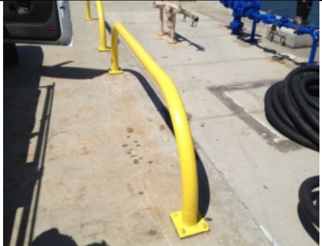
Guard rail, painted yellow; Pt. Loma Subase
