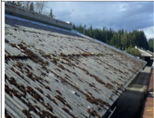
Roof, (via gutter); Bangor
