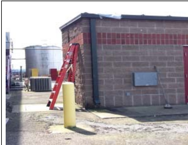
Shed roof, green coated metal; NAVSTA Everett
