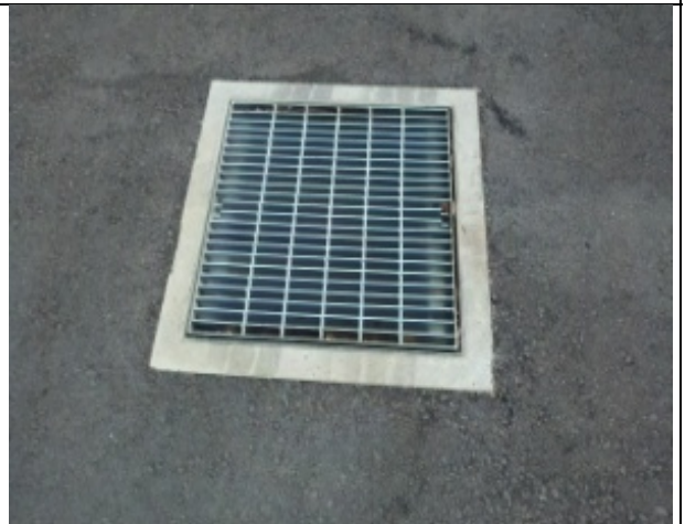
Grate 2, stormwater drain; NBSD
