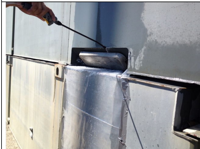
Causeway, portion with zinc anode; Little Creek
