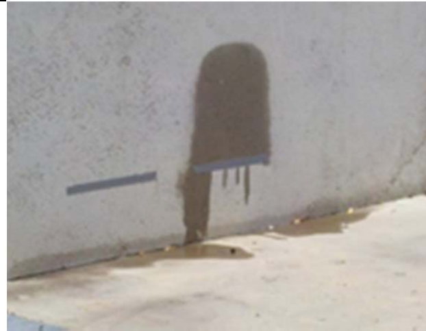
Concrete wall; SSC-PAC
