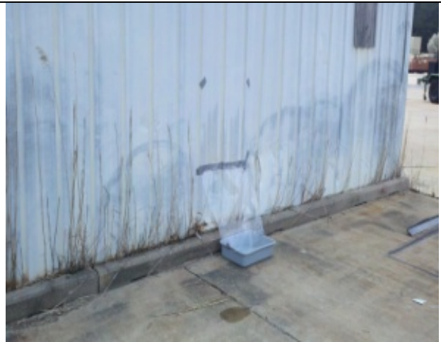
Metal panel, painted galvanized, building side; Saint Julian
