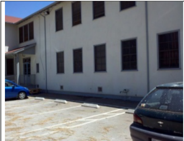
Plaster wall, painted white; SSC-PAC
