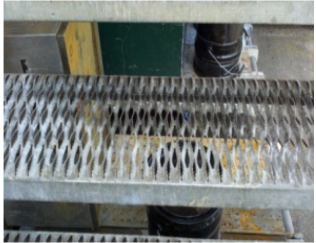
Figure 50: Galvanized stairs, grating
