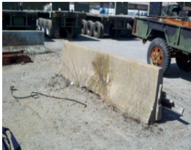
Figure 11: Concrete barrier, uncoated
