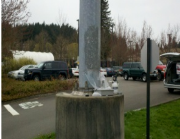
Figure 53: Utility pole, galvanized
