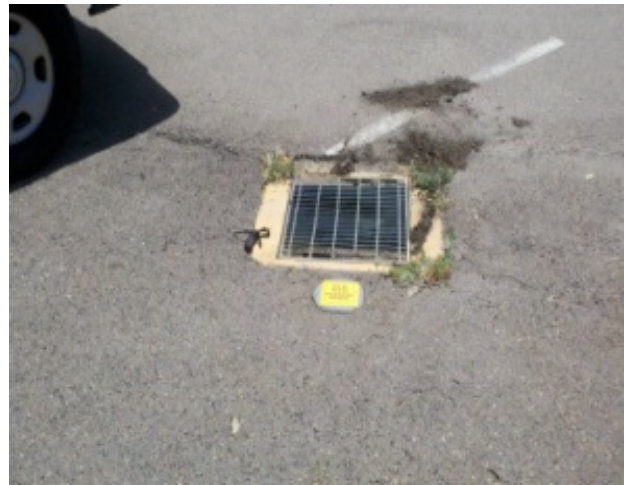
Figure 32: Grate, stormwater drain
