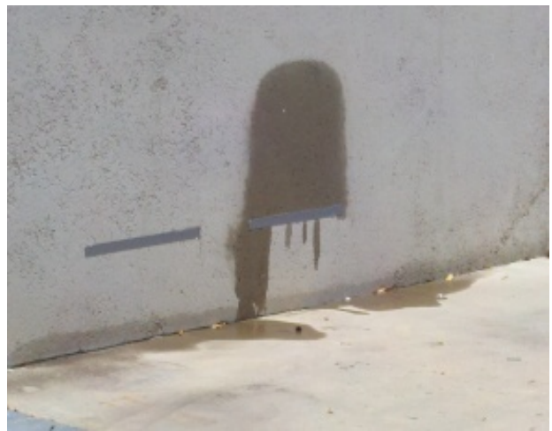
Figure 12: Concrete wall, uncoated
