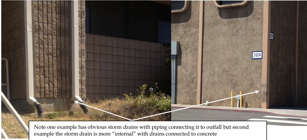
Figure 17. Examples of "direct" connect buildings with runoff directly to outfall drainage system.
