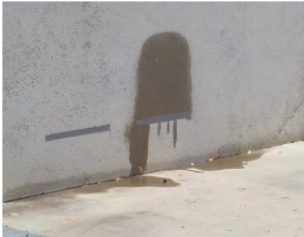
Figure 13: Concrete wall, coated, gray
