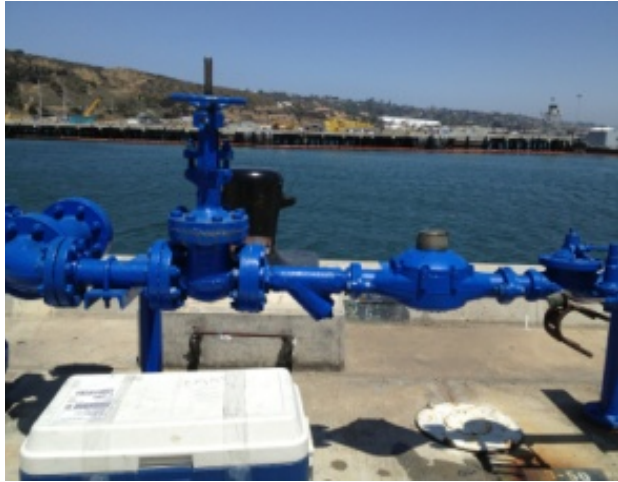
Figure 57: Water riser, potable, blue (w/brass)
