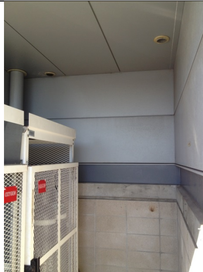
Bldg. 633 southwest corner roof drains
