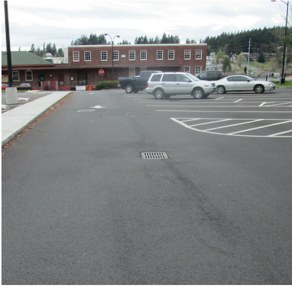
Figure 9. Examples of street and parking areas directly connected to the conveyance system (left) and indirectly connected through a vegetated swale.
