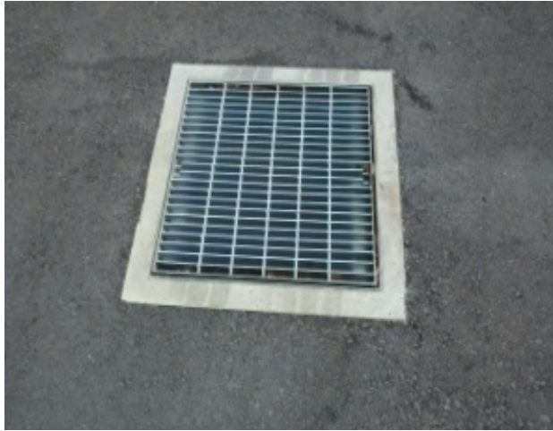
Figure 33: Grate, stormwater drain
