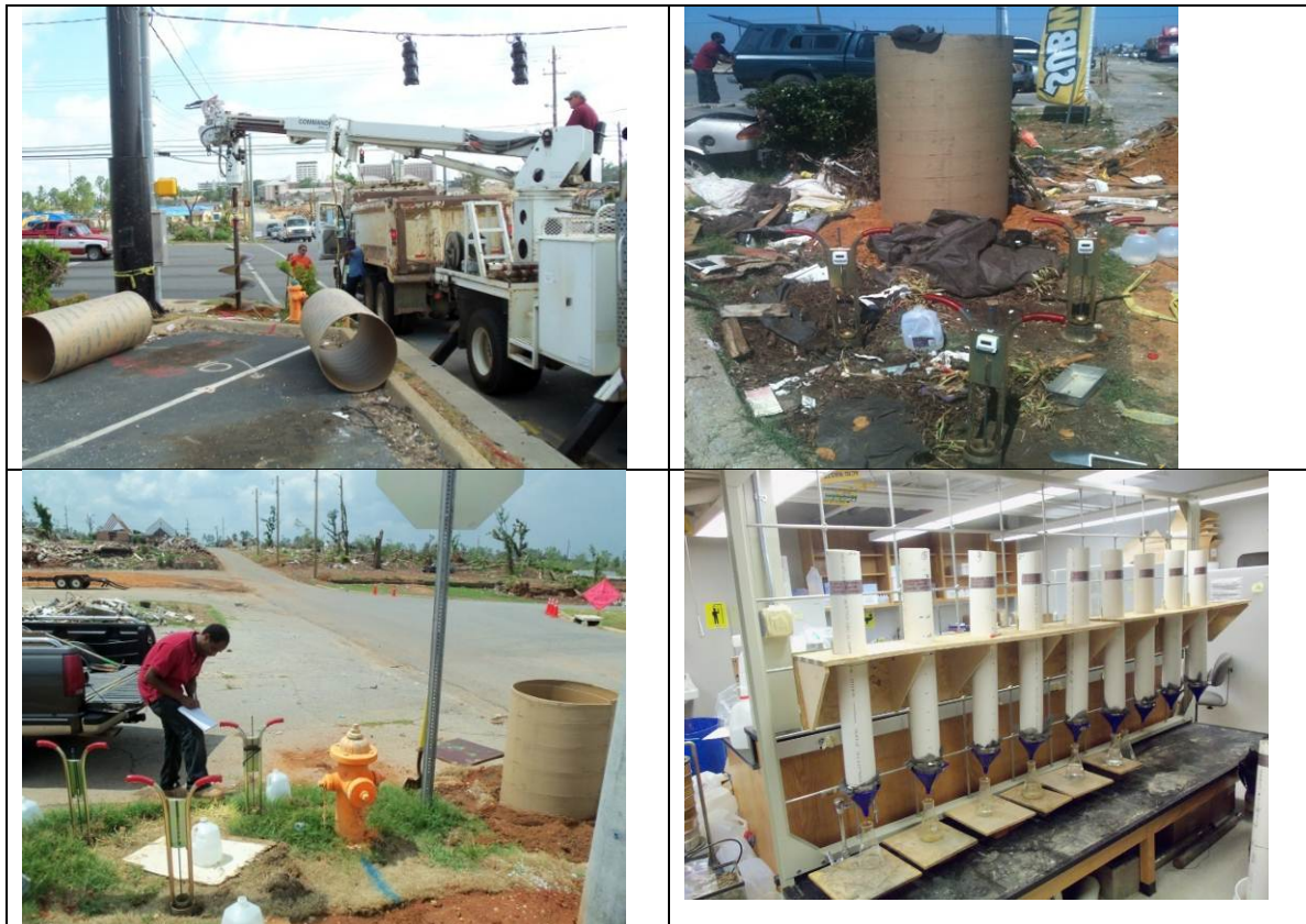
Figure 3. Photographs showing borehole drilling, Sonotube infiltration tube installation, double-ring infiltration measurements, and laboratory column tests.
