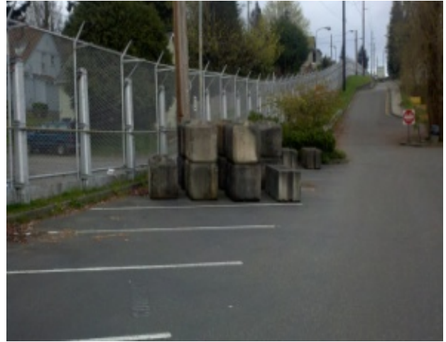
Figure 22: Fence, galvanized, painted
