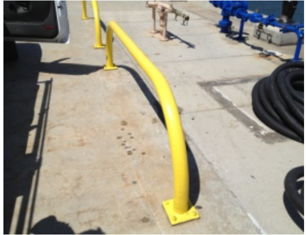
Figure 34: Guard rail, painted, yellow
