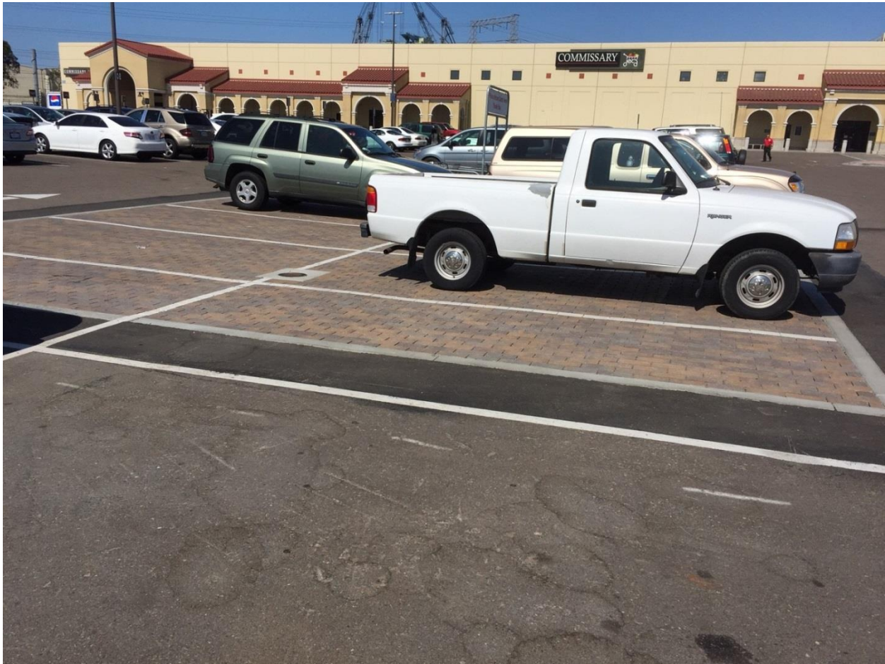
Figure 11. View of completed Paver site facing north. The cart return in the upper middle of the photo is roughly in the middle of the site and over the top of the main stormwater conveyance overflow drain.
