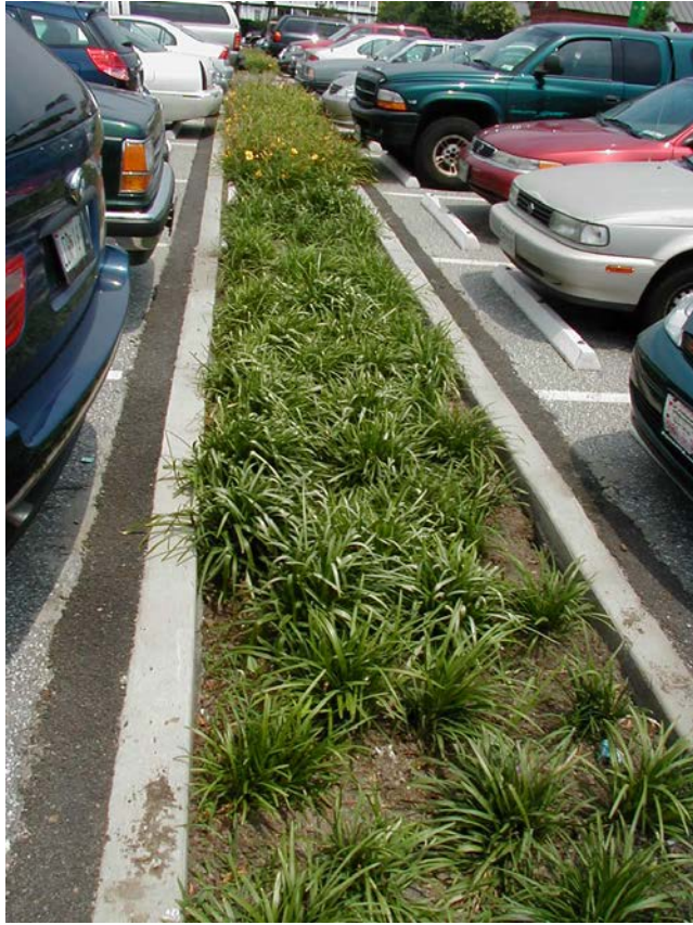
Figure 3-14: Navy Yard Bioretention
