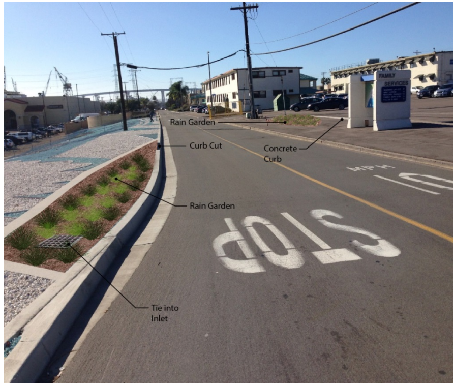
Figure 3-21: LID Pilot Project Site 3 Concept Design Schematic
