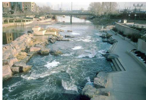
Figure 2.14 Cherry Creek and Platte River junction in Denver, CO.
