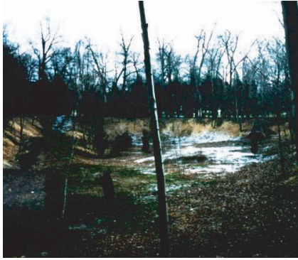
Figure 3.11 Groundwater recharge basin in Long Island, NY, using stormwater. (Courtesy of New York Department of USGS).
