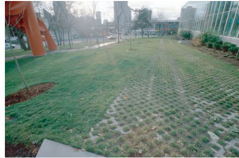
Figure 3.16 Paver blocks for occasional access road, Seattle Science Center, WA.
