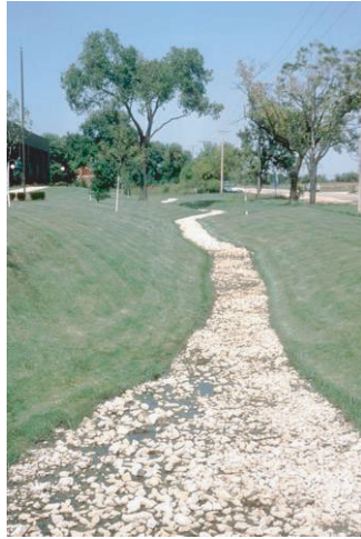
Figure 3.19 Stormwater infiltration through infiltration trench, office park, Lake Oswego, OR.
