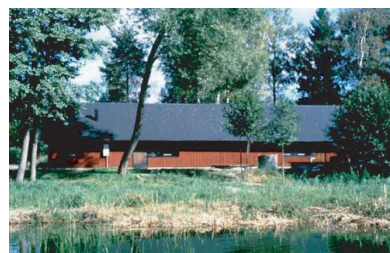
Figure 4.26 Chemical treatment facility at FBM installation at Lake Rönningesjön, Sweden. (Used with permission of Fresh Creek Technologies, Inc.)
