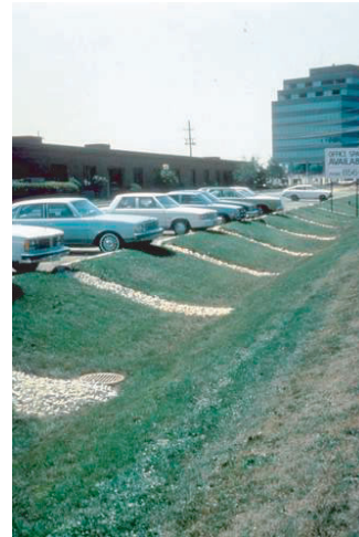
Figure 3.18 Grass swale in office park area, Milwaukee, WI.
