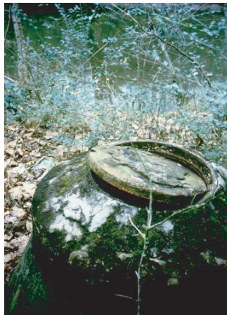
Figure 4.46 Typical SSO discharge point along banks of Five-Mile Creek.
