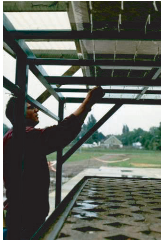
Figure 6.33 Adjustments being made to rain drop tubes at Essen infiltration test apparatus.
