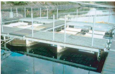
Figure 3.25 TrashTrap™ at Fresh Creek, Brooklyn, NY.
