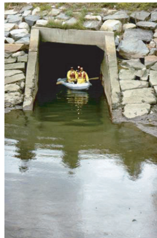
Figure 6.117 Manual surveys conducted in Boston in large tidally influenced storm drains.
