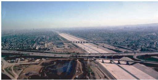
Figure 4.39 Los Angeles River and roadway crossings.
