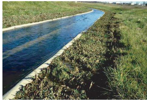
Figure 3.9 Lined channel in Milwaukee, WI.
