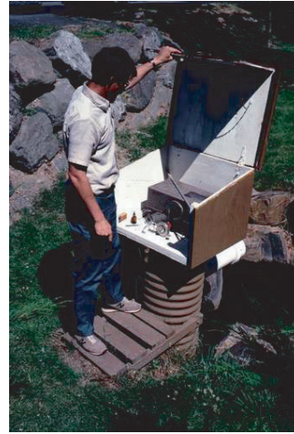
Figure 4.20 Level recorder at Bellevue flow monitoring station.
