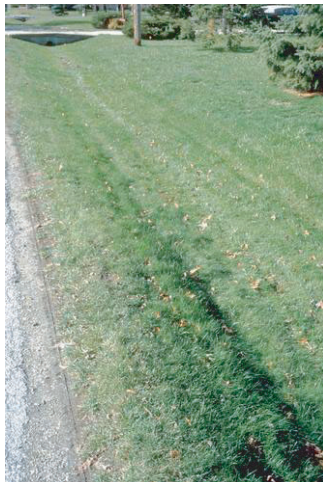
Figure 3.17 Grass swale in residential area, Milwaukee, WI.
