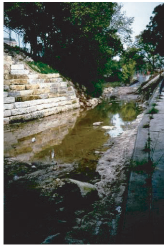
Figure 3.8 Lined embankment along Waller Creek, Austin, TX.
