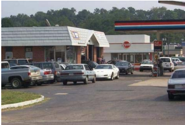
Paved parking area with frequent automobile movement
