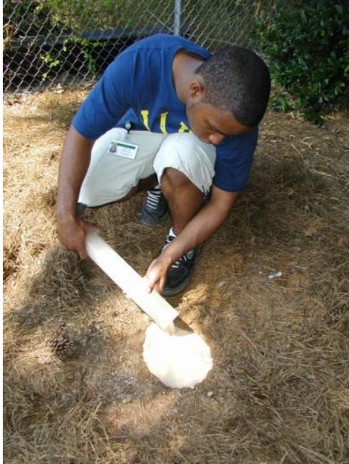
Direct soil density measurement; filling excavated hole with sand.
