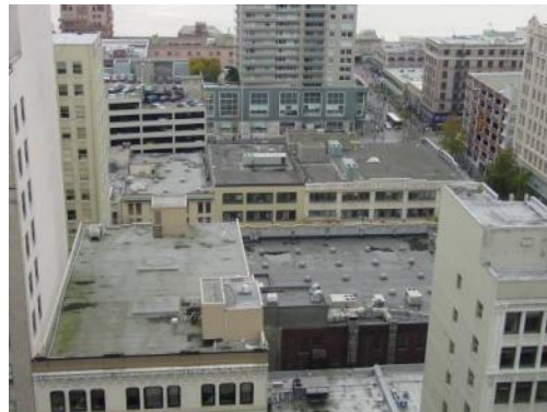
Flat commercial roofs
