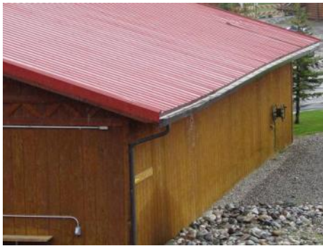
Pitched metal roof
