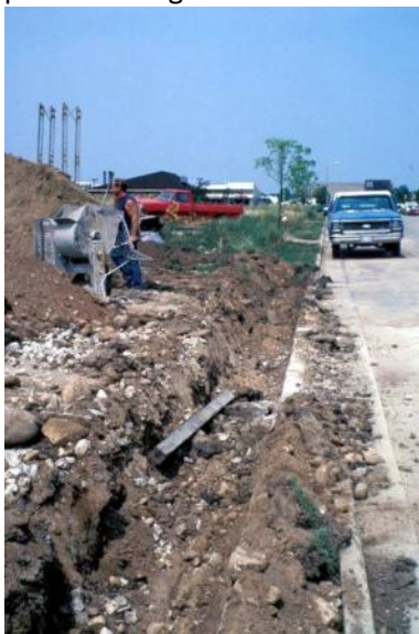
Utility work near street.
