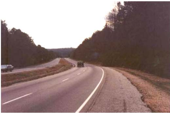
Suburban freeway with large shoulders and grass swales at median
