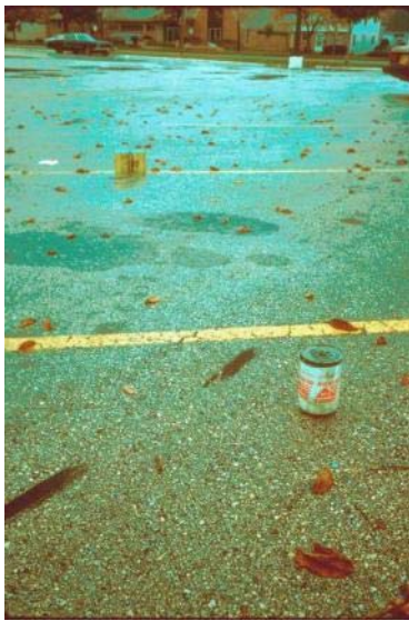
Contamination of paved parking area due to inappropriate waste disposal
