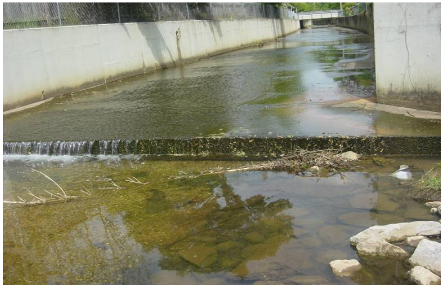
Figure 6-36. Concrete channel along Cribbs Mill Creek
