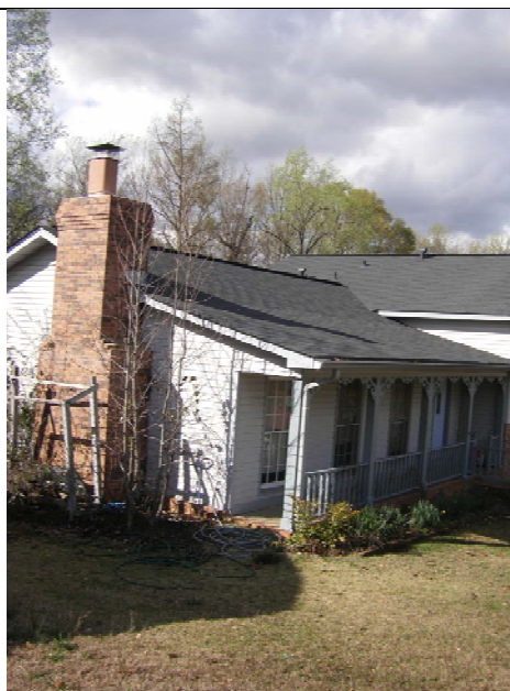
Residential roof sampling location
