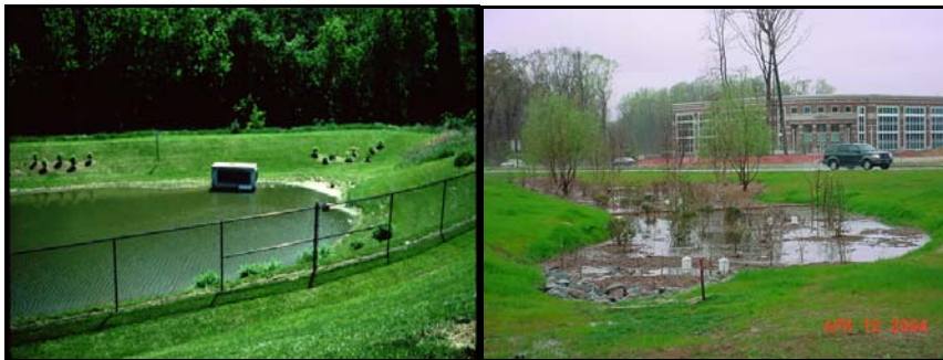
Figure 1. a) Simple STP monitoring situation – defined single inlet and single outlet of a wet pond; b) complex STP monitoring situation – multiple inlet locations, evapotranspiration and infiltration losses at a bioretention facility
