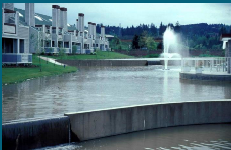
Apartments, Lake Oswego, OR (Part of Treatment Train)
