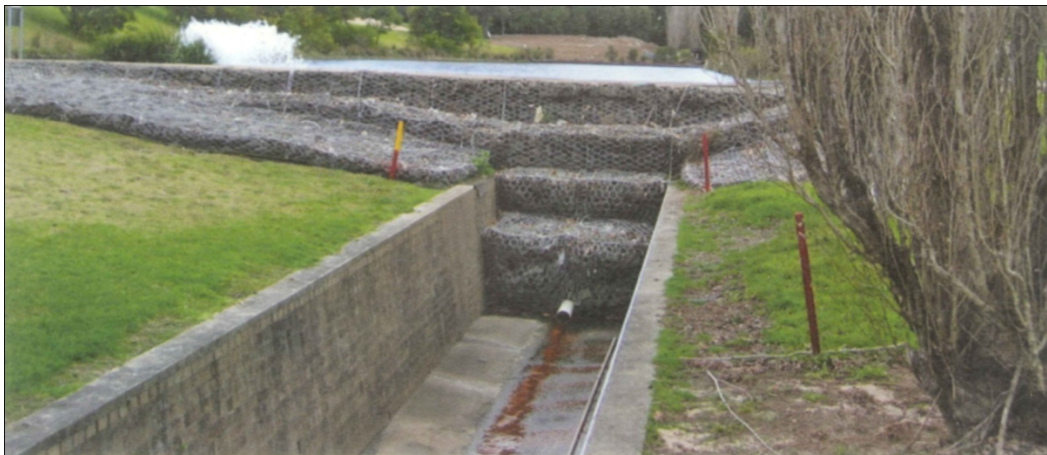
Figure 3-8. Bexley Stormwater Harvesting Project. (Source: 2006 NSW Metropolitan Water Plan) (Used by permission of www.environment.nsw.gov.au )
