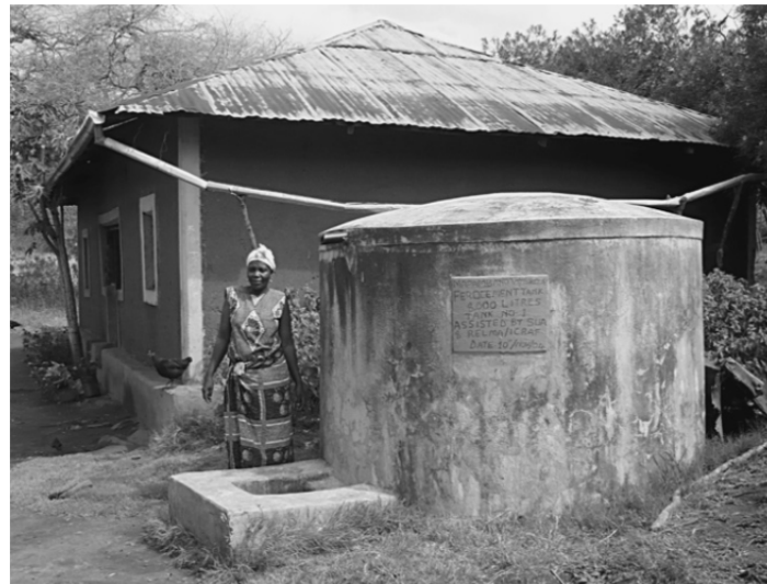
Figure 3-4. Rooftop Rainwater Harvesting Tank. (Reprinted from Agricultural Water Management, 9 (2010), Pachpute, J. S., A package of water management practices for sustainable growth and improved production of vegetable crop in labour and water scarce Sub-Saharan Africa, pp. 1251-1258, 2010, with permission from Elsevier)
