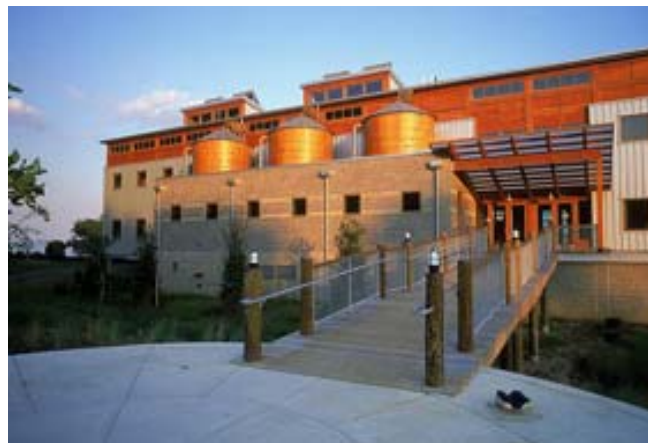
Figure 3-11. Exterior North view and Rainwater Harvesting Tanks in Philip Merrill Building, Annapolis. ( http://www.nrel.gov/buildings/pdfs/34830.pdf )
