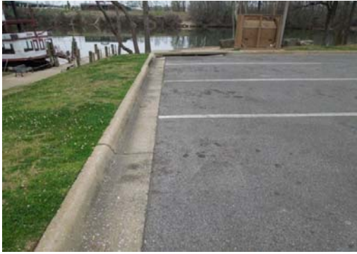
Runoff enters filter inlet through roadside gutter and pavement sheetflow
