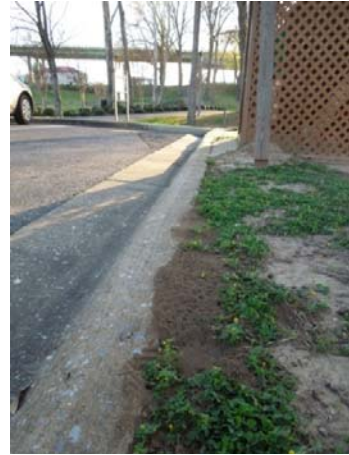
Fire ant hills besides the filter inlet increased the sediment load into the filter during some storms due to erosion
