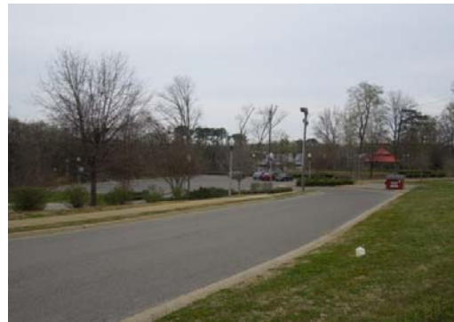
Slight slope along the parking lot entrance road directs the runoff into the parking area and filter
